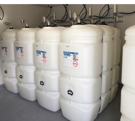
OEL TANK LAGER
